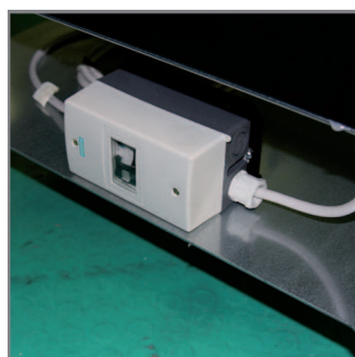
Quadro comandi Electric panel board
